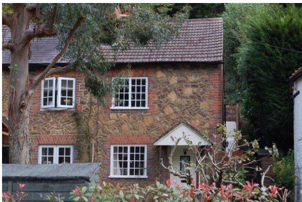
Figure 8: Creative stonework typical of late Victorian architects (105 Brighton Road).
